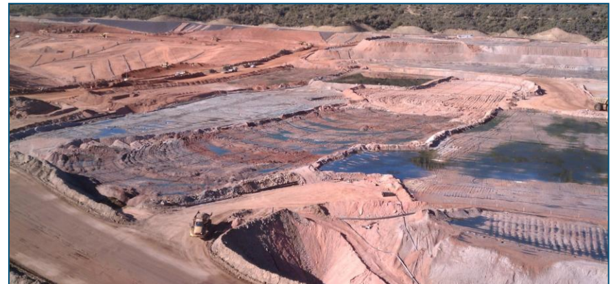
Transition to Conveyor Stacking
