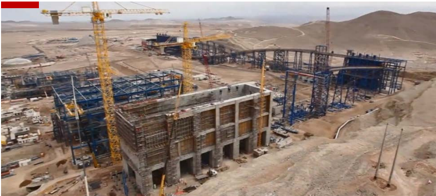
▪ Milled ore warehouse
