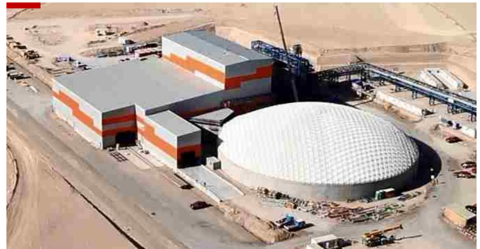
Cu concentrate filtration installation
