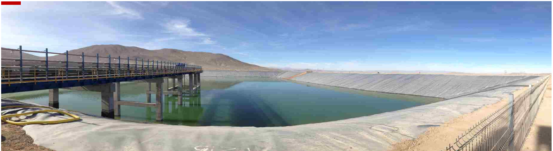
Sea water reservoir with capacity 750 thousand m 3
