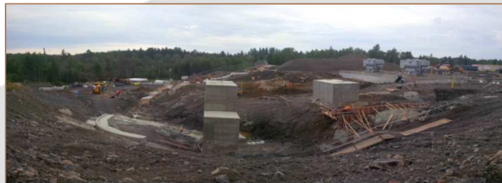
Foundations of the 230 kV transformer station
