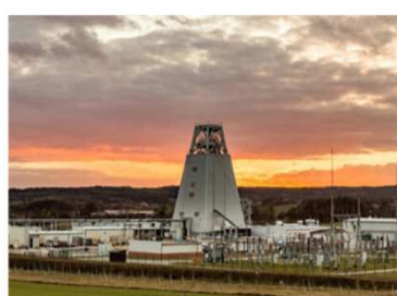
GG-1 shaft sinking site
