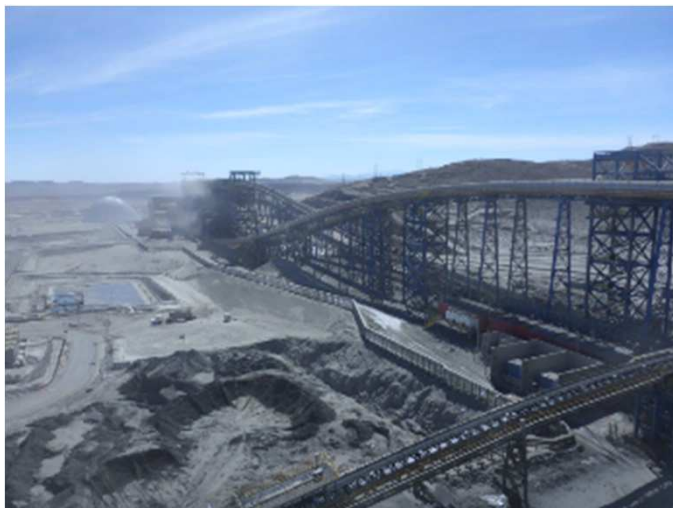
Ore processing at the Sierra Gorda mine
