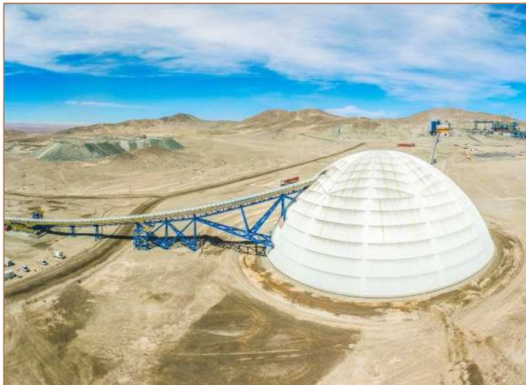
Coarse ore stockpile facility
