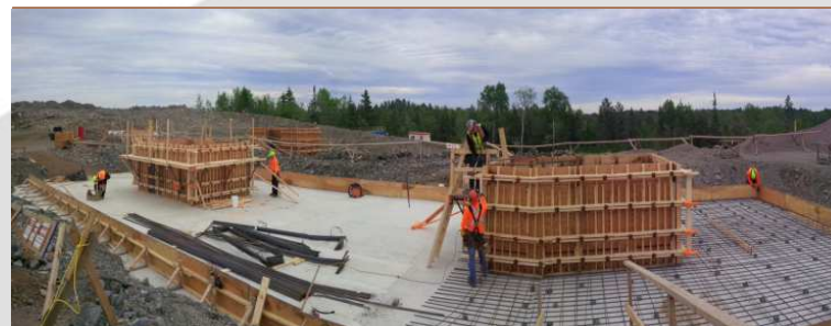
Foundations of the 230 kV transformer station
