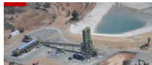
Application of new tailings storage technology (paste technology)
