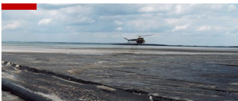
Development of the Żelazny Most tailings pond
