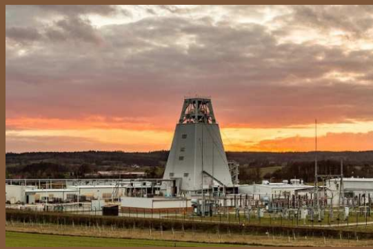
Worksite of GG-1 shaft
