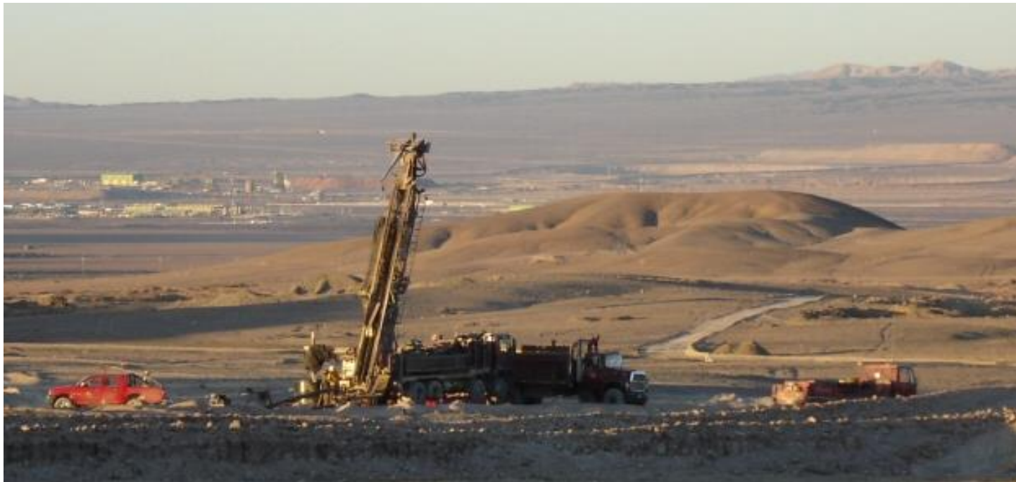
Drilling rig in the Pampa Lina exploration zone
