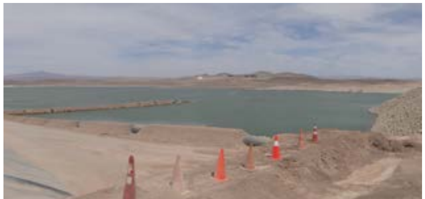
Tailings storage facility - Sierra Gorda, Chile
