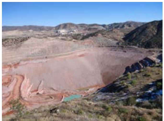
Buttress supporting the Pinto Creek Diversion Channel - Carlota mine, Arizona, USA
