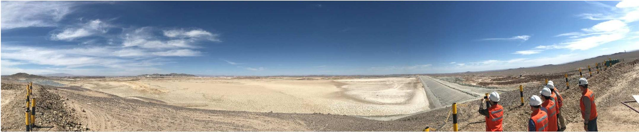
In recent months Sierra Gorda has been working on ensuring the proper functioning of the tailings storage facility and securing further waste storage capability. Due to the low content of solids in waste and the accumulation of water in the storage facility, a potential risk of reduced facility stability has been identified.
