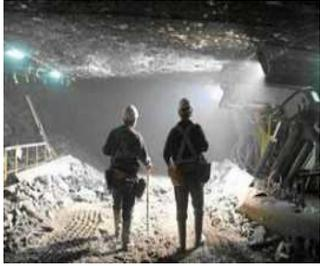
The **DAP Program** includes the construction of the **GG-1 ventilation shaft** designed for transporting material and employees, with a target depth of 1350m and a diameter of 7.5m.
